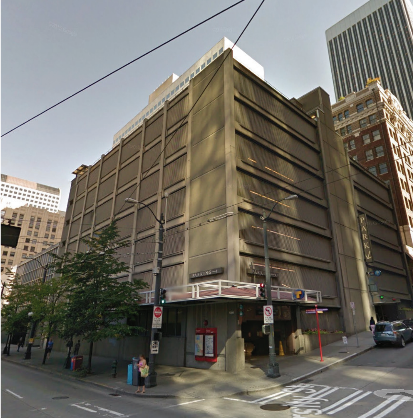
fig. 33 1300 3rd Ave. existing condition
