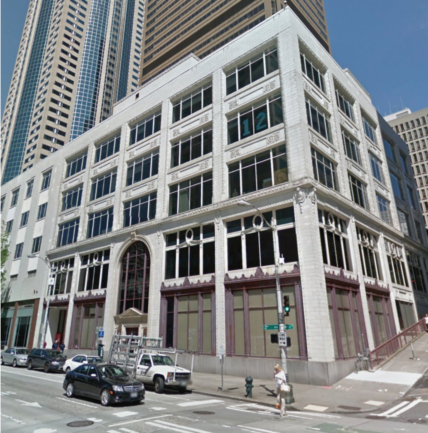
fig. 39 1100 2nd Ave. existing condition
