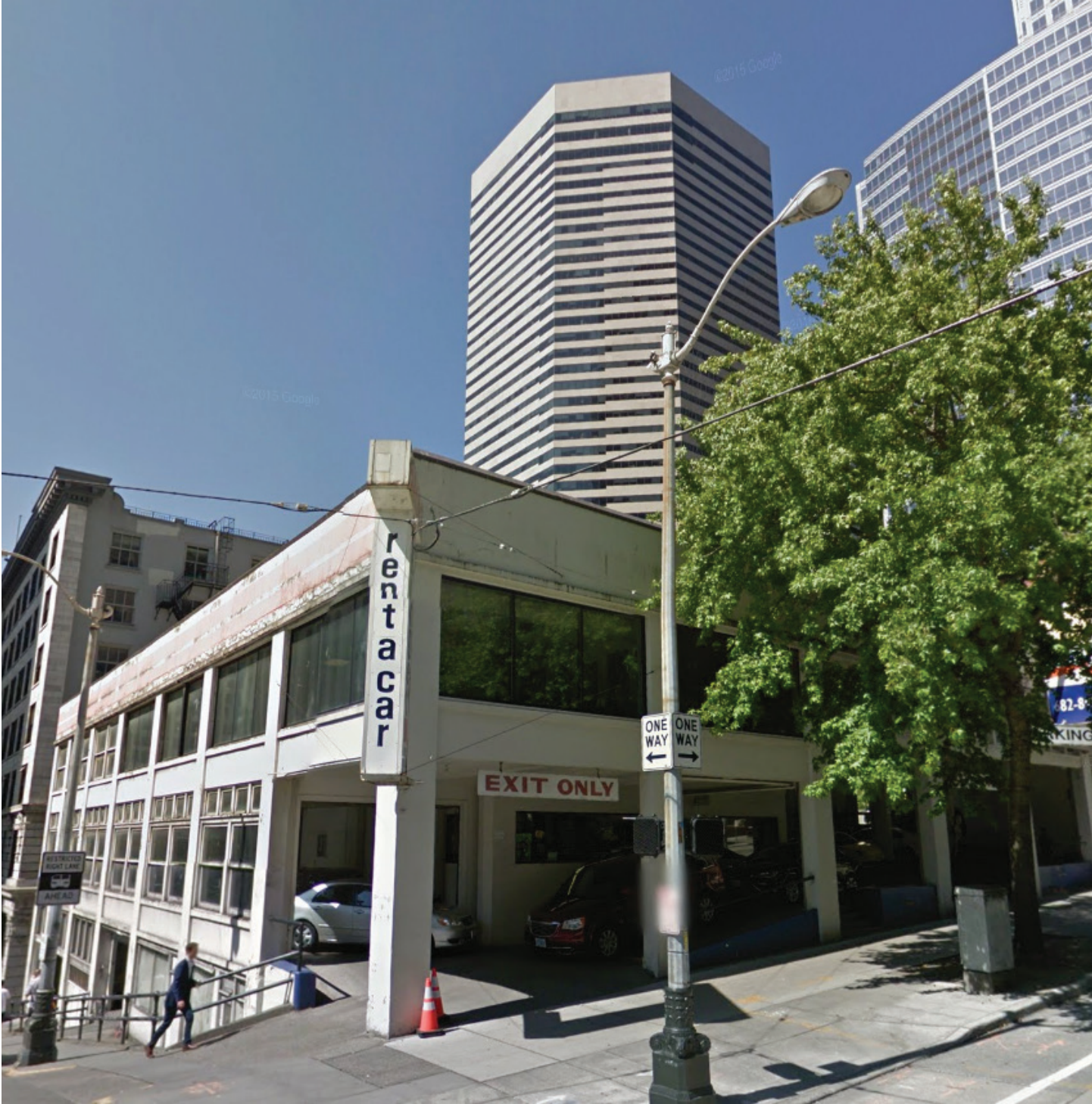
fig. 37 807 4th Ave. existing condition
