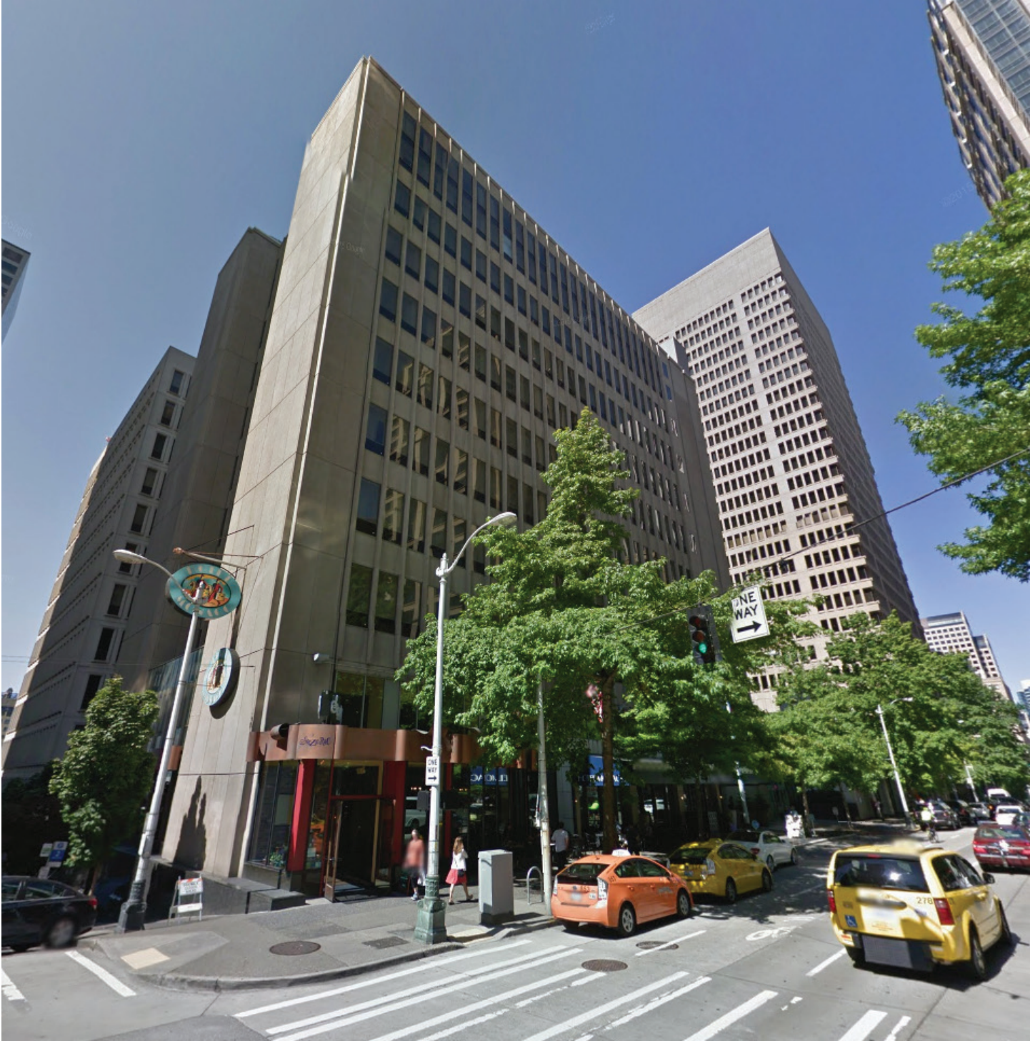
fig. 35 1101 4th Ave. existing condition
