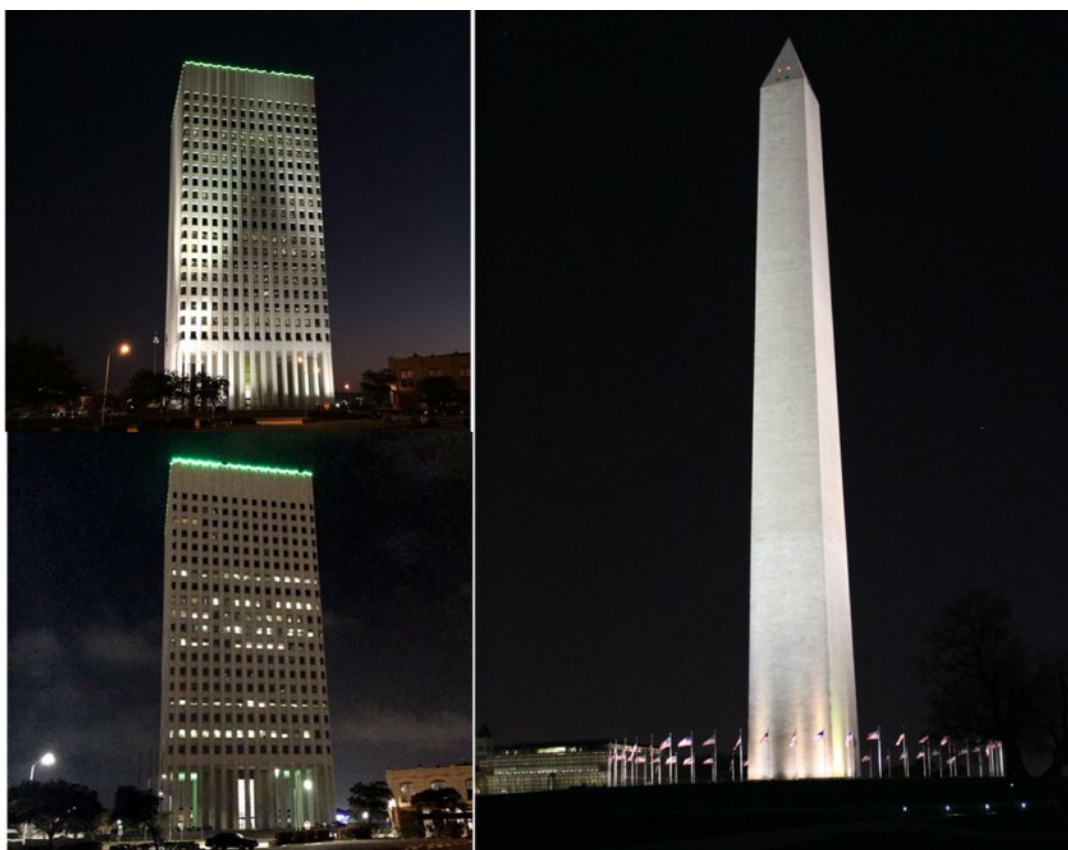
Figure 16. Dangerous Floodlights: One Moody Plaza and The Washington Monument Left: One Moody Plaza with flood lights on (top) and off (bottom). Right: The Washington Monument showing a floodlit structure and two red warning lights. pollution, a floodlit structure, and two red warning lights.
