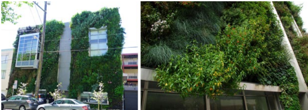
Figure 7. Green Wall on the Sam Cuddleback III Assembly Wing, San Francisco, CA
