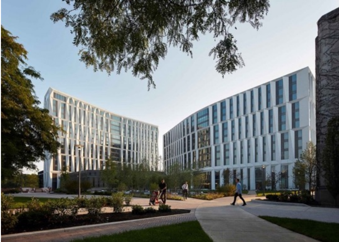
Figure 34. University Of Chicago Campus North Residential Commons
