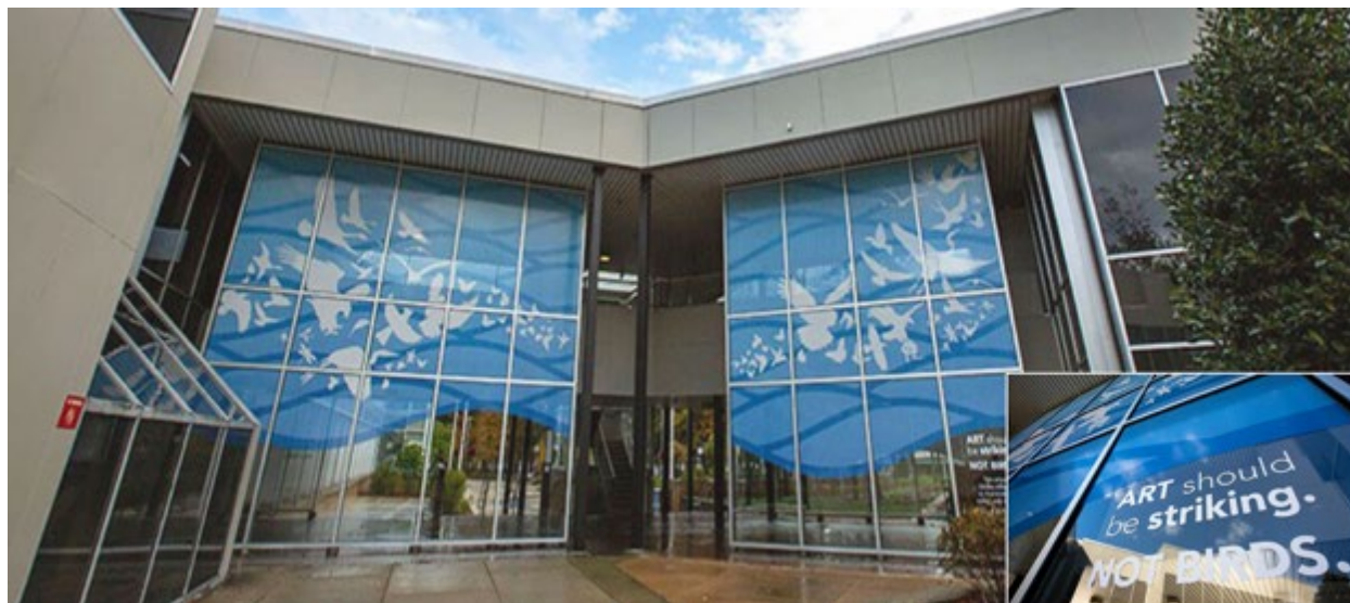
Figure 38. Perforated Vinyl on the Stockton University K-Wing Building
