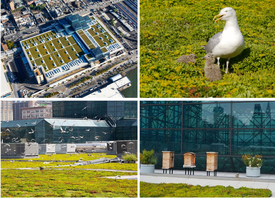
Figure 30. Jacob Javits Convention Center Green Roof Left Top and Bottom: Javits Convention Center Green Roof. Right Top: Herring gull ( Larus argentatus ) Family. Right Bottom: Glass Façade and Beehives.
