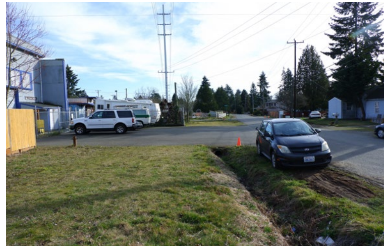
Figure A.4 Block 3 stormwater swale
