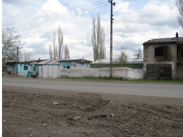
Figure 4.16: The built environment around Kars Museum, May 2010 (Photograph was taken by the author.)
