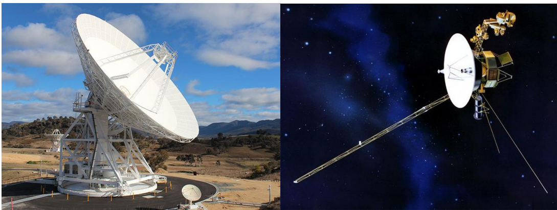
Figure 2.9: Deep Space Network 34m dish antenna (left), Voyager spacecraft with a 4m dish antenna (right)
