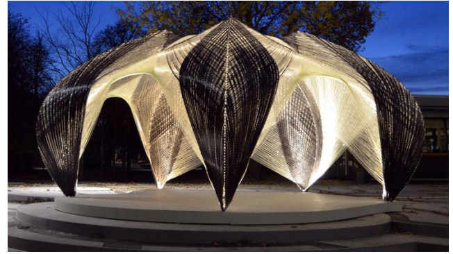
fig. 23 Monocoque carbon and glass fiber shell
