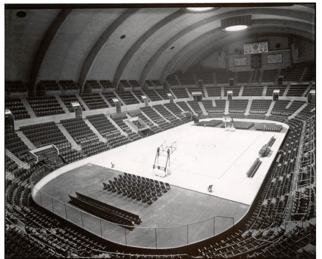
fig. 5 Stiffeners supporting shell, Hershey Arena built 1936
