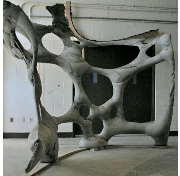
fig. 17 Structure created with adjustable formwork
