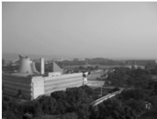
Figure 21: The Capitol Complex, Landmark Site
