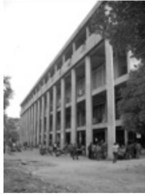
Figure 22: Contributing Modern Structure
