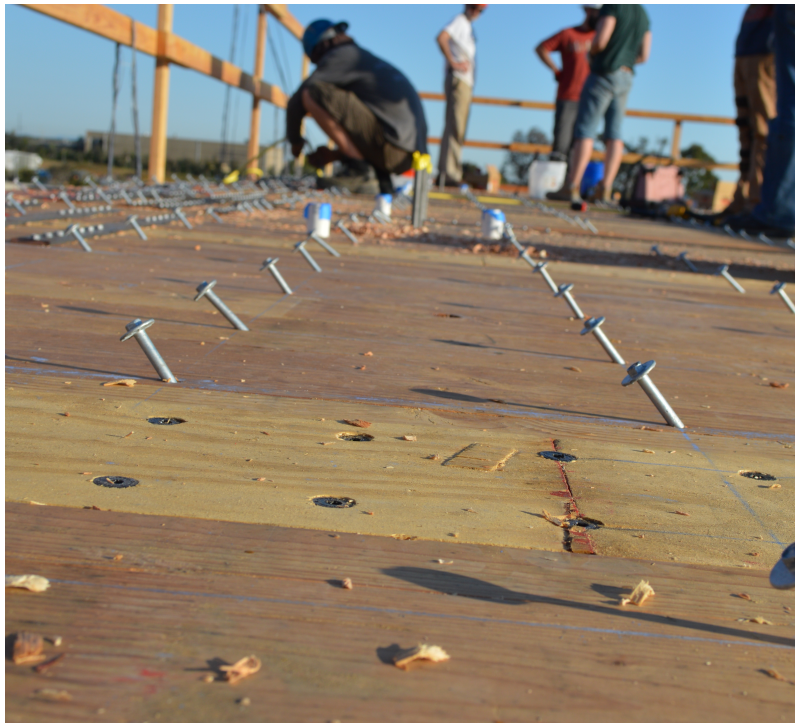
Figure 4.12: Shear screws used for CLT concrete composite deck on the roof
