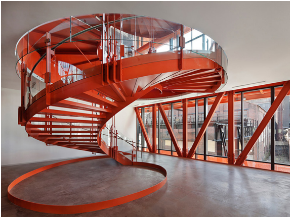
Figure 27. Steel spiral staircase
