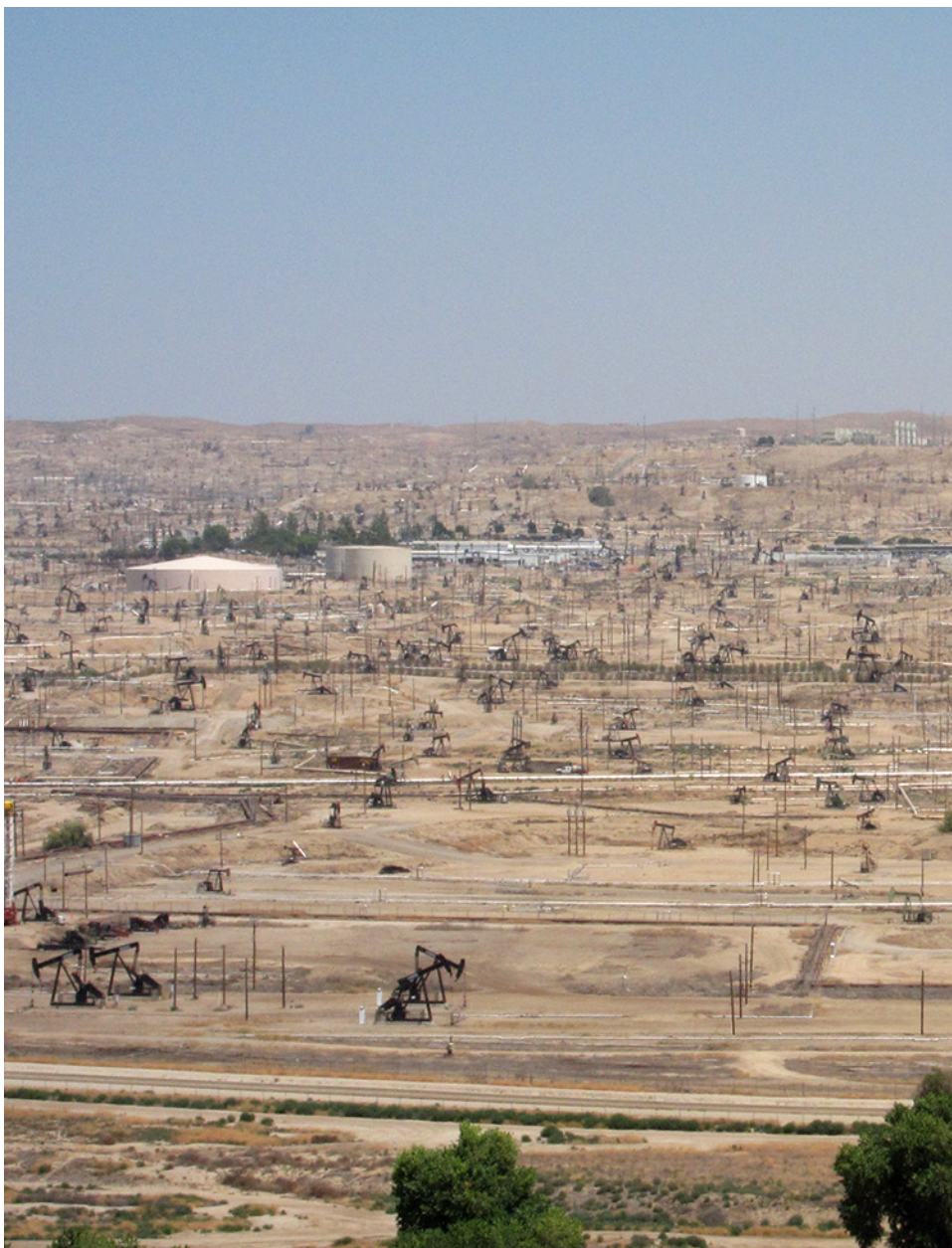
Figure 34. View facing north of Kern River Oil Field with storage tanks and cogeneration plant visible
