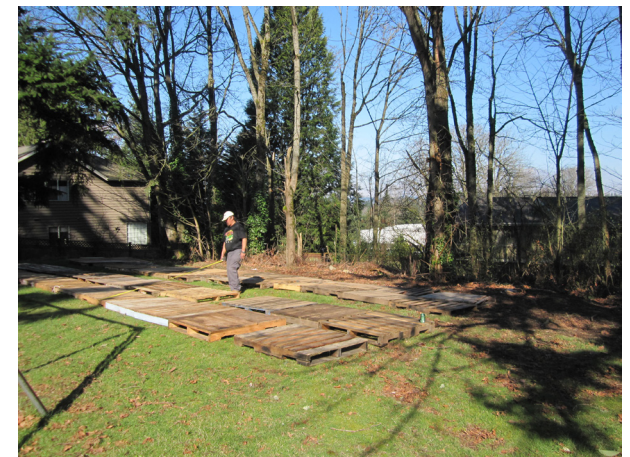
FIGURE 32. Laying Out Pallets.
