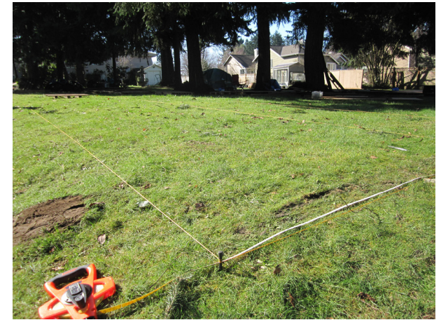
FIGURE 31. Laying String Lines for the New Campsite.
