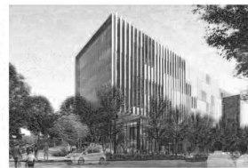
④ POPULATION HEALTH BUILDING (UNDER CONSTRUCTION)
