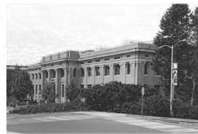
② ARCH HALL
