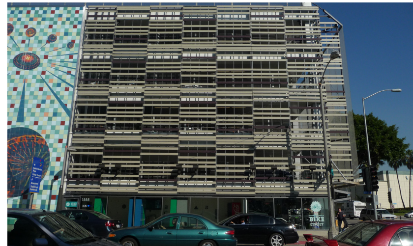
Figure 30 Exterior of Santa Monica Bike Center integrated with a parking garage. Jessica Lass, Make Biking to Work your 2012 resolution, switchboard.nrdc.org , Web.
