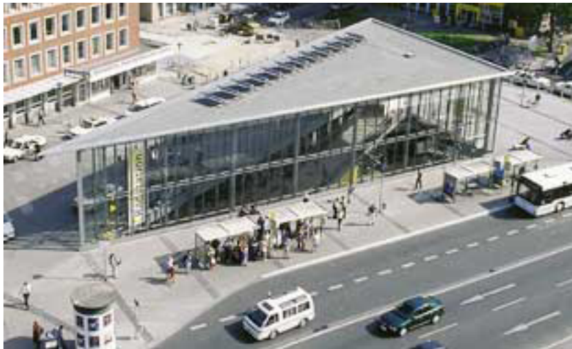
Figure 35 Radstation from above. At street level it has a glass facade and the bicycle parking is below. Stadt Muenster, "Die Radstation," www.muenster.de , Web.
