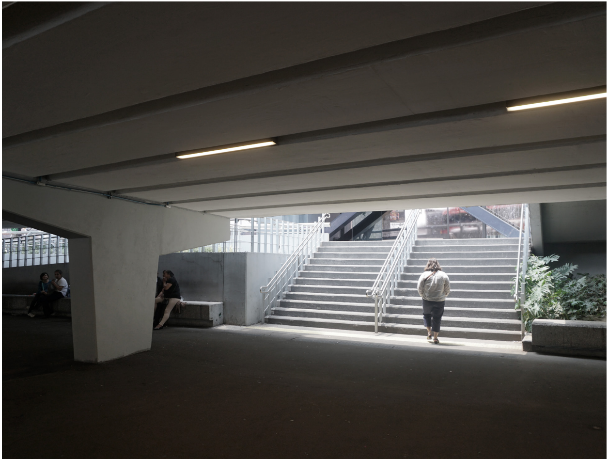
fig. 32 Pedestrian access to Ministry of Public Security
