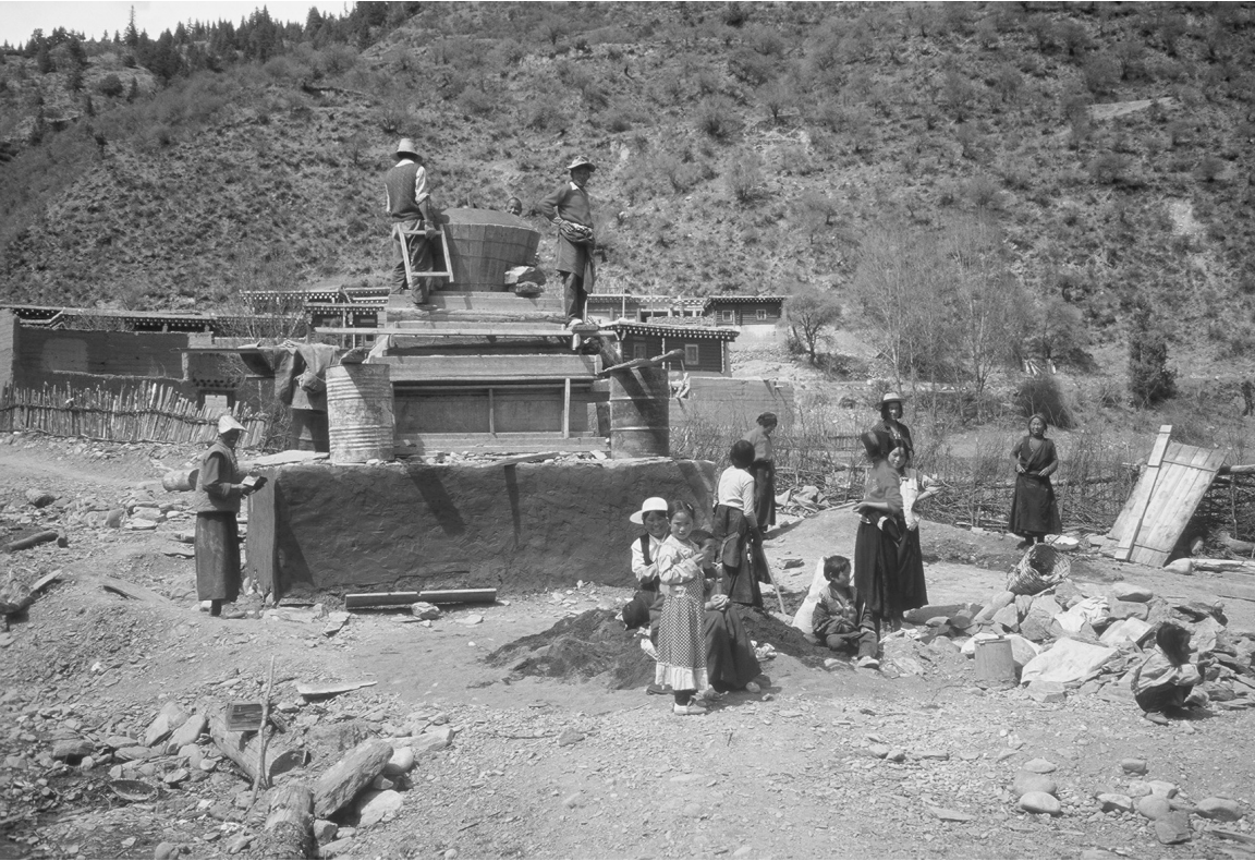
FIG. 2.9. Villagers in Drango County, Kandze, working on a new stupa.
