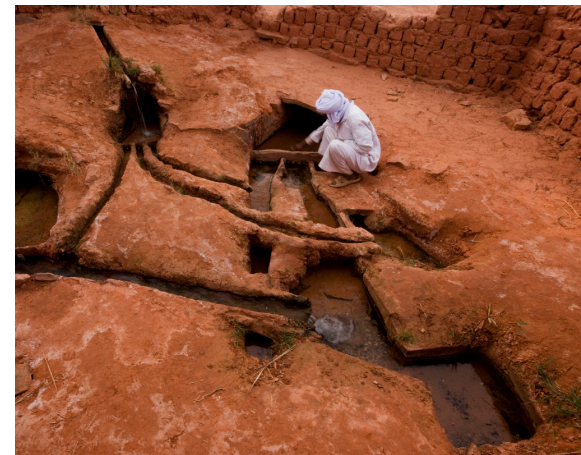
Figure 3.10. Earthen water meter directing water to different stakeholders and locations. Beni Isguen, Algeria. Source: George Steinmetz.
