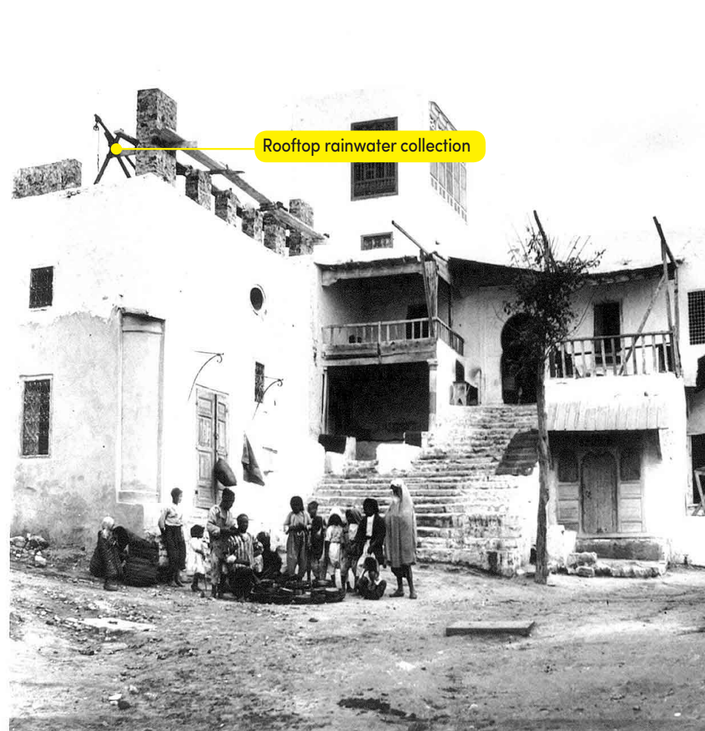
Figure 2.11. Evidence of rooftop water harvest on a house in Sidi Bou Said, north of the city of Tunis. 1889.
