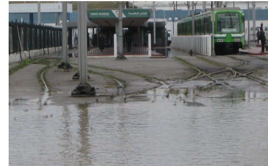
Figure 2.18. Flooded TGM metro station in downtown Tunis following rain in November 2012. Source: Robin Worldwide
