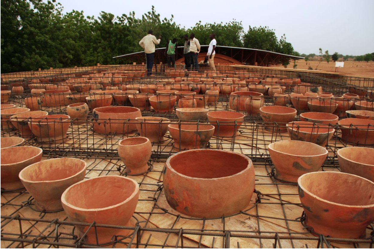
Figure 26: Gando School Library Roof Under Construction
