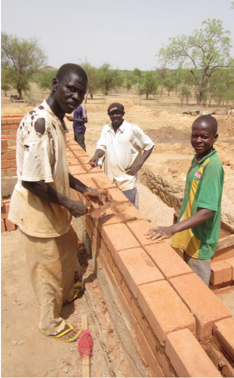
Figure 17: (top) Opera Village Construction Crew Members
