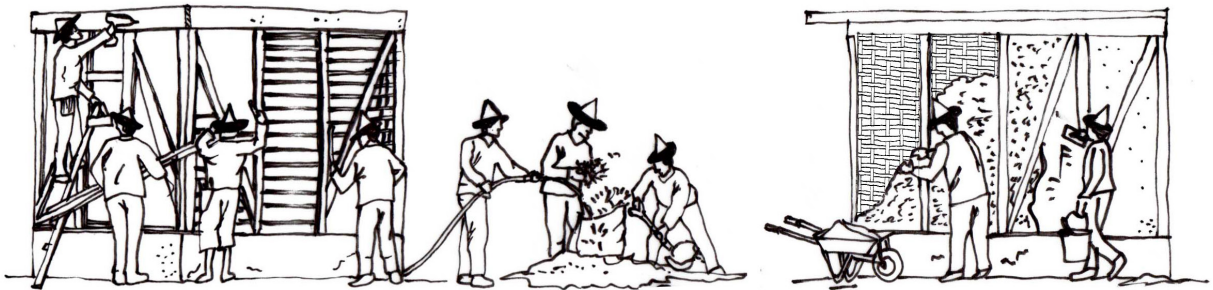
Figure 8: Wattle and Daub building technique. Similar to BASE methodology except BASE uses Bamboo over timber framing.
