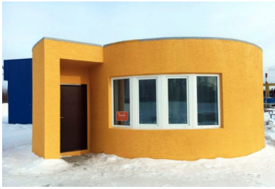
a) Example of non-engineered 3D printed structure
