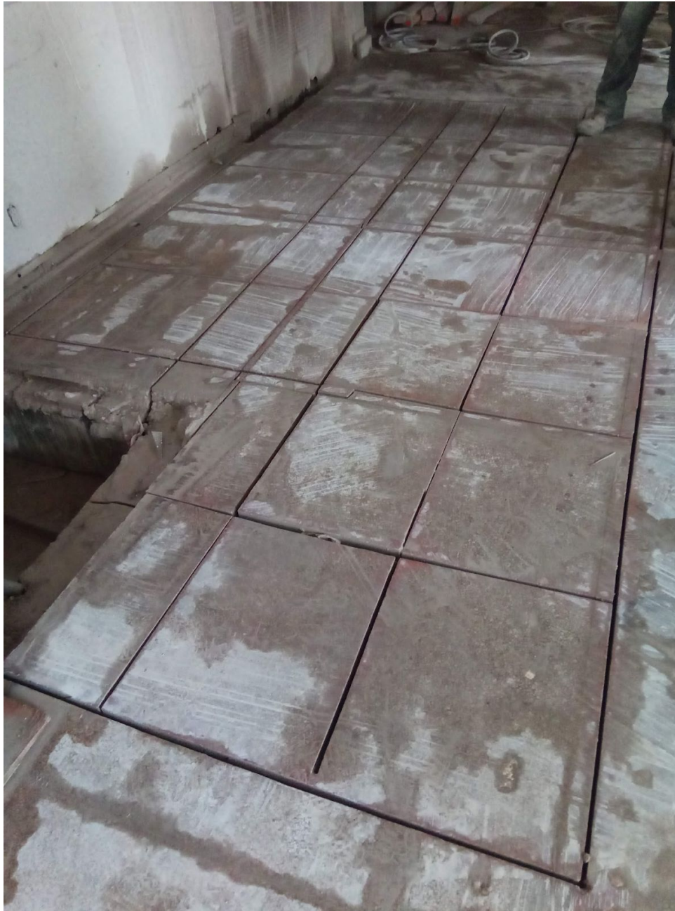
Figure 11: Remnants of water used while sawcutting
