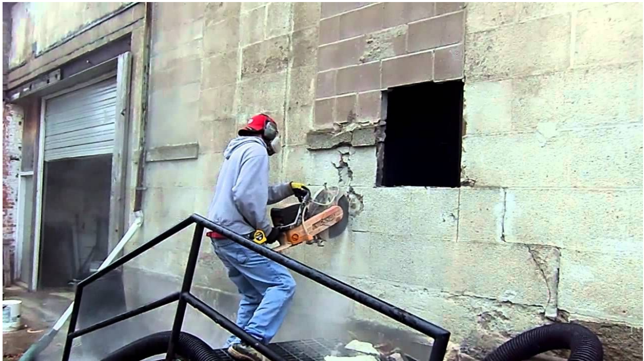
Figure 12: Demolition saw being used to demolish a concrete/CMU wall (Televideo, 2011).
