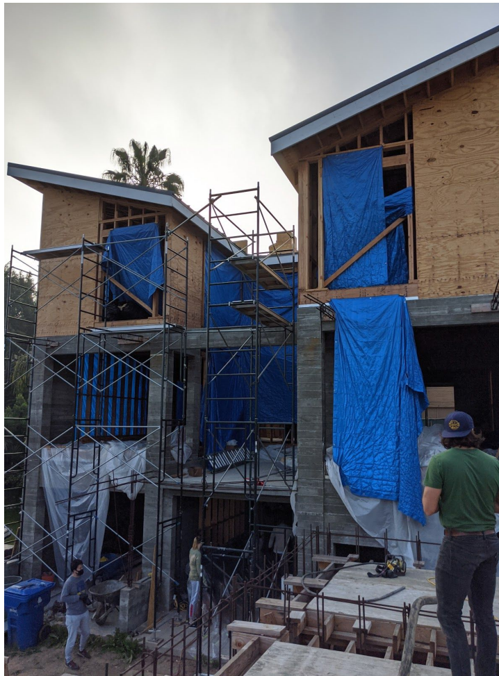
Figure 6: Concrete Walls in Los Angeles
