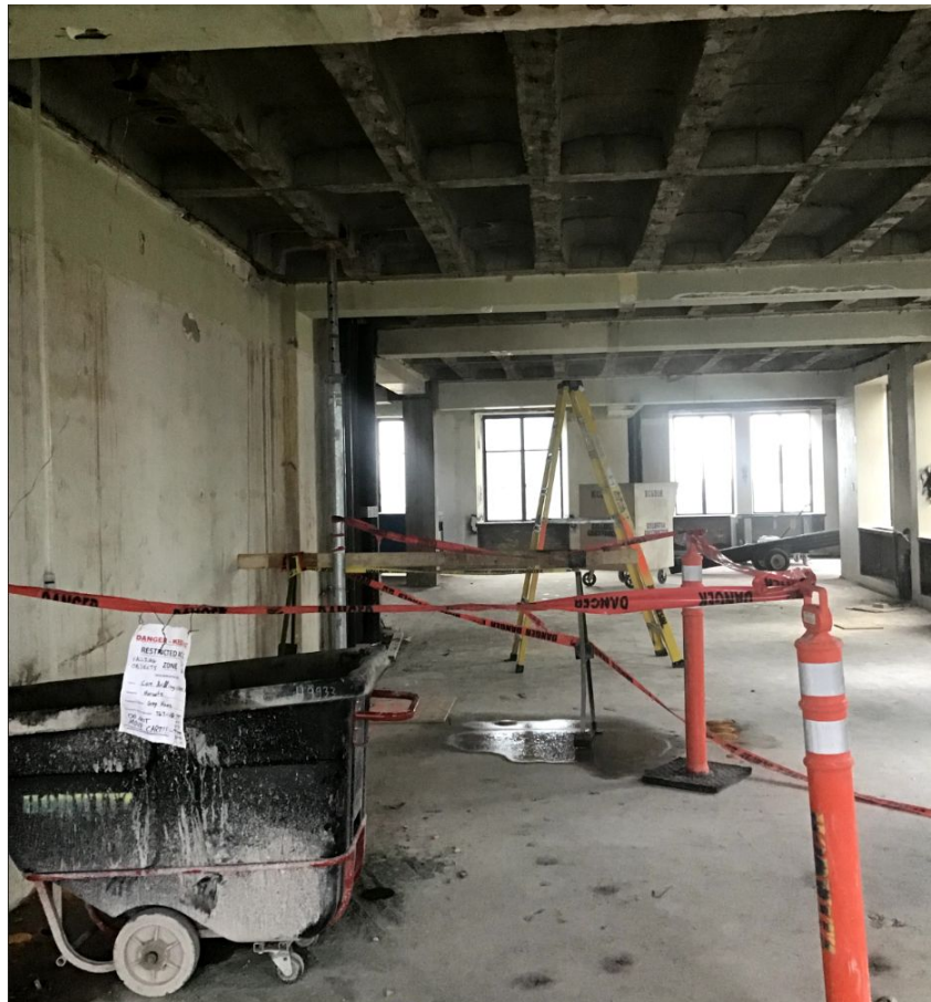
Figure 10: Water suppression used during core drilling.
