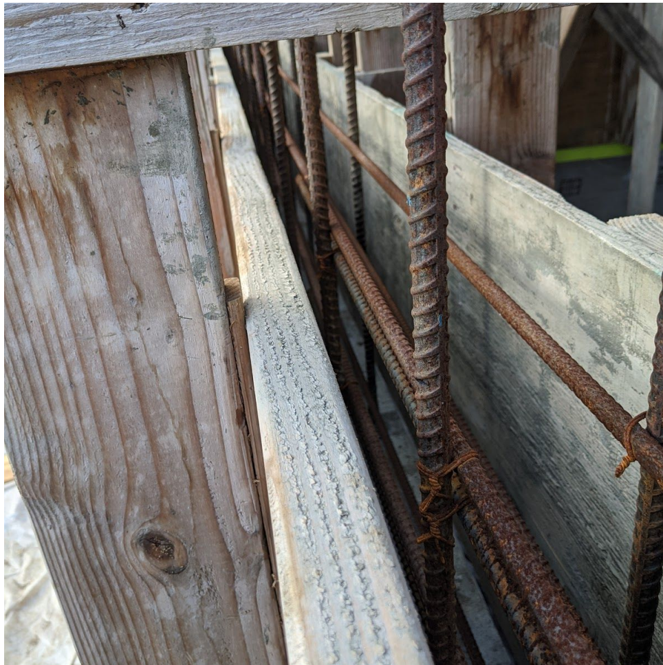
Figure 7: Reused Concrete Form Boards, Scraped
