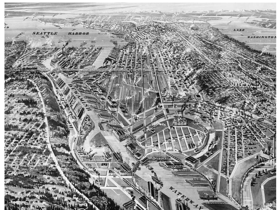
fig. 6 Dredging the Duwamish, 1922 fig. 7 Island as a Machine
