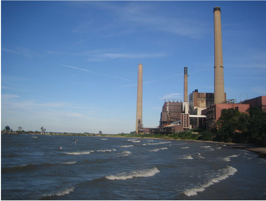
A coal-fired power plant located near Cleveland, OH.
