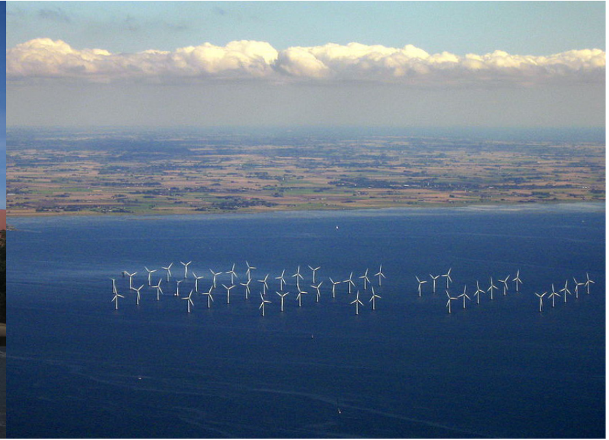
Overwater Wind Farm in Sweden
