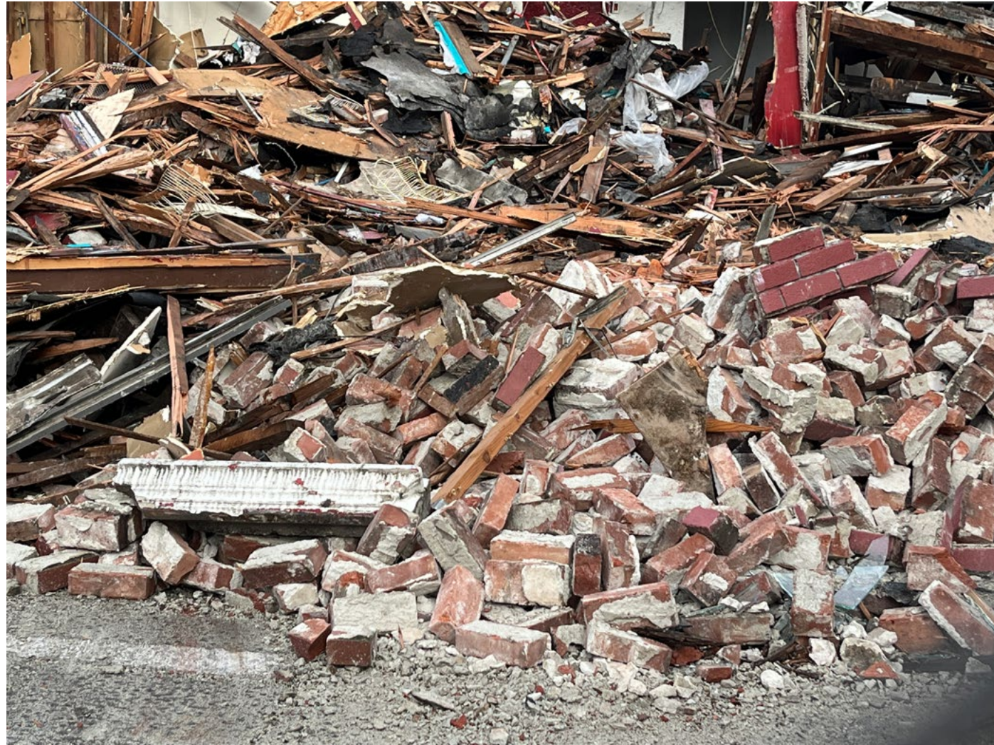
Figure 6.4 Materials piled on site prior to landfilling
