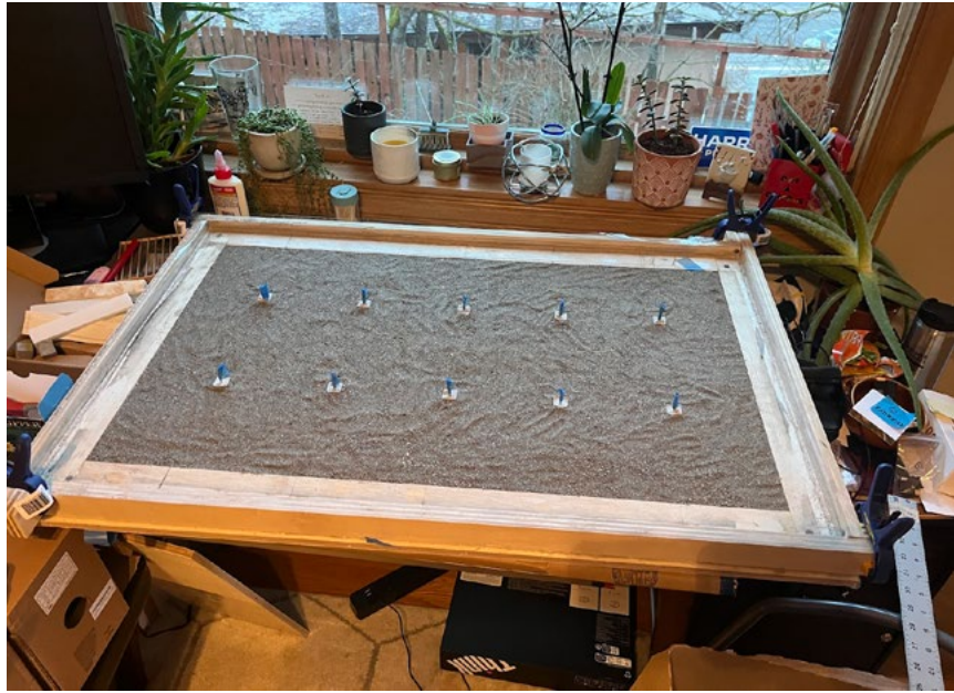
Sand acts as aggregate, keeping footers in place prior to pouring of concrete slab.
