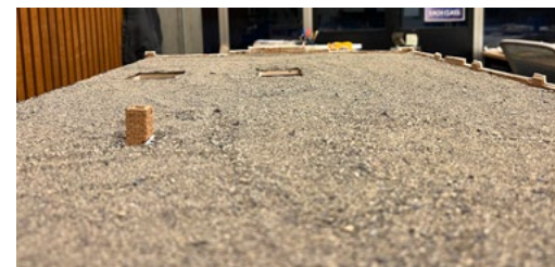
Roof: wood base, fabric paper and asphalt-based roof coating, gravel
