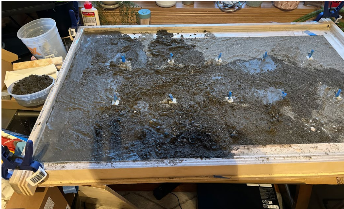
Concrete mix failure.
