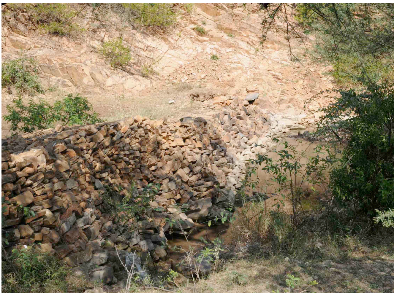
Stones slanting upwards: a bund that works with the movement of water in a stream course
