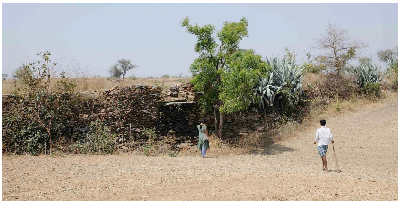
A stone bund with waste weir: layers of stone stacked over generations
