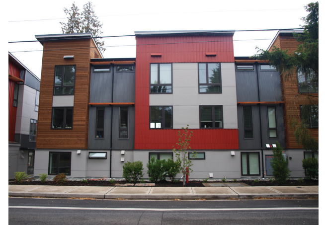
Fig. 56. Rental apartment street facade.
