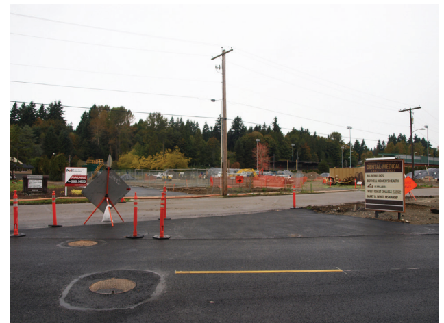
Fig. 91. View of site from 98th Avenue NE.
