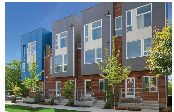
Fig. 27. Seattle, WA: Townhouse development by B9 Architects. (Photo credit: B9 Architects)
