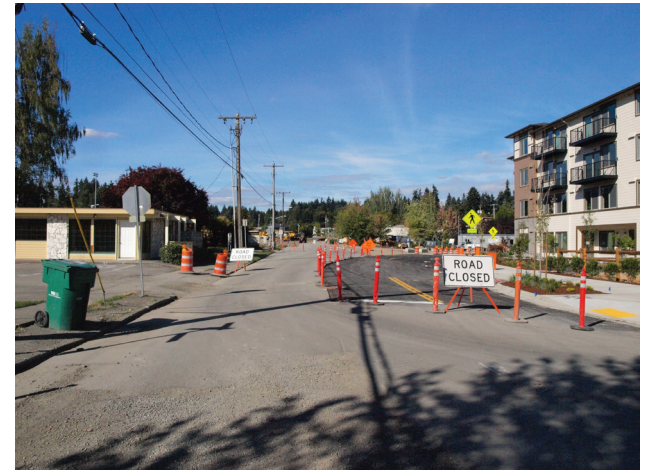
Fig. 90. View up 98th Avenue NE.
