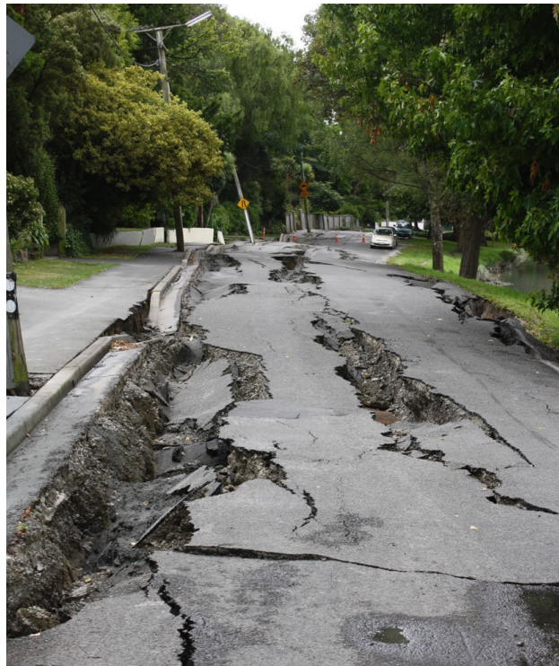
Figure 2.22: Ground cracks in pavement on a residential street, due to liquefaction-induced lateral spreading in the 2011 Christchurch Earthquake (Wikipedia Commons)
