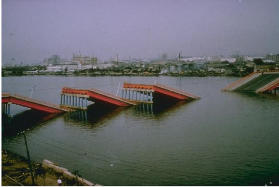
Figure 2.3: Collapse of simply supported deck sections of the Showa Bridge in Niigata city, due to ground shaking and liquefaction from the 1964 Niigata Earthquake (U.S. Geologic Survey)
