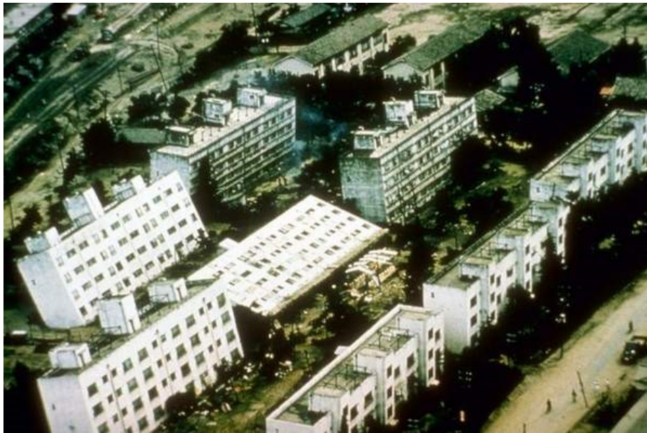
Figure 2.2: Collapse of a series of apartment buildings in Niigata city due to liquefaction-induced bearing failure from the 1964 Niigata Earthquake (U.S. Geologic Survey)
