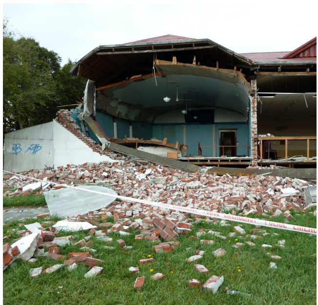
4: Piles of rubble in the earthquake aftermath
