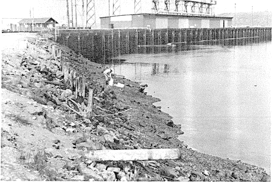
Figure 2. Photograph taken 8 April 1985 of Slip 1 beach looking to west. The tide level is +0.7 m. Note the irregular waterline caused by the pits and peaks of the beach.
