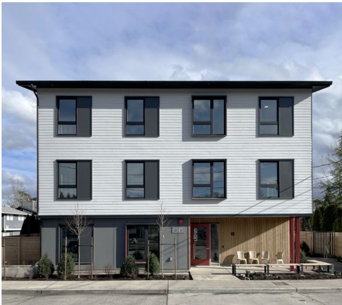
Figure 7. Photograph of Red Willow Residences in Seattle, WA, a 12-unit Passive House certified apartment building with a unique investment structure to improve affordability (VY Architecture 2024).
