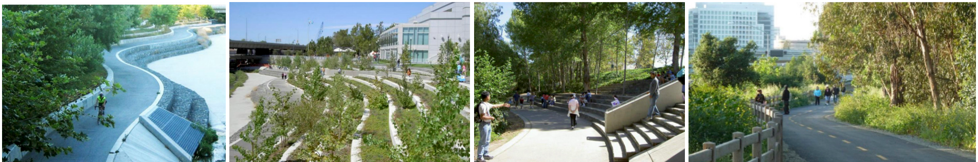
Figure 21. Gabion wall system and terraces for protecting the riverbank
