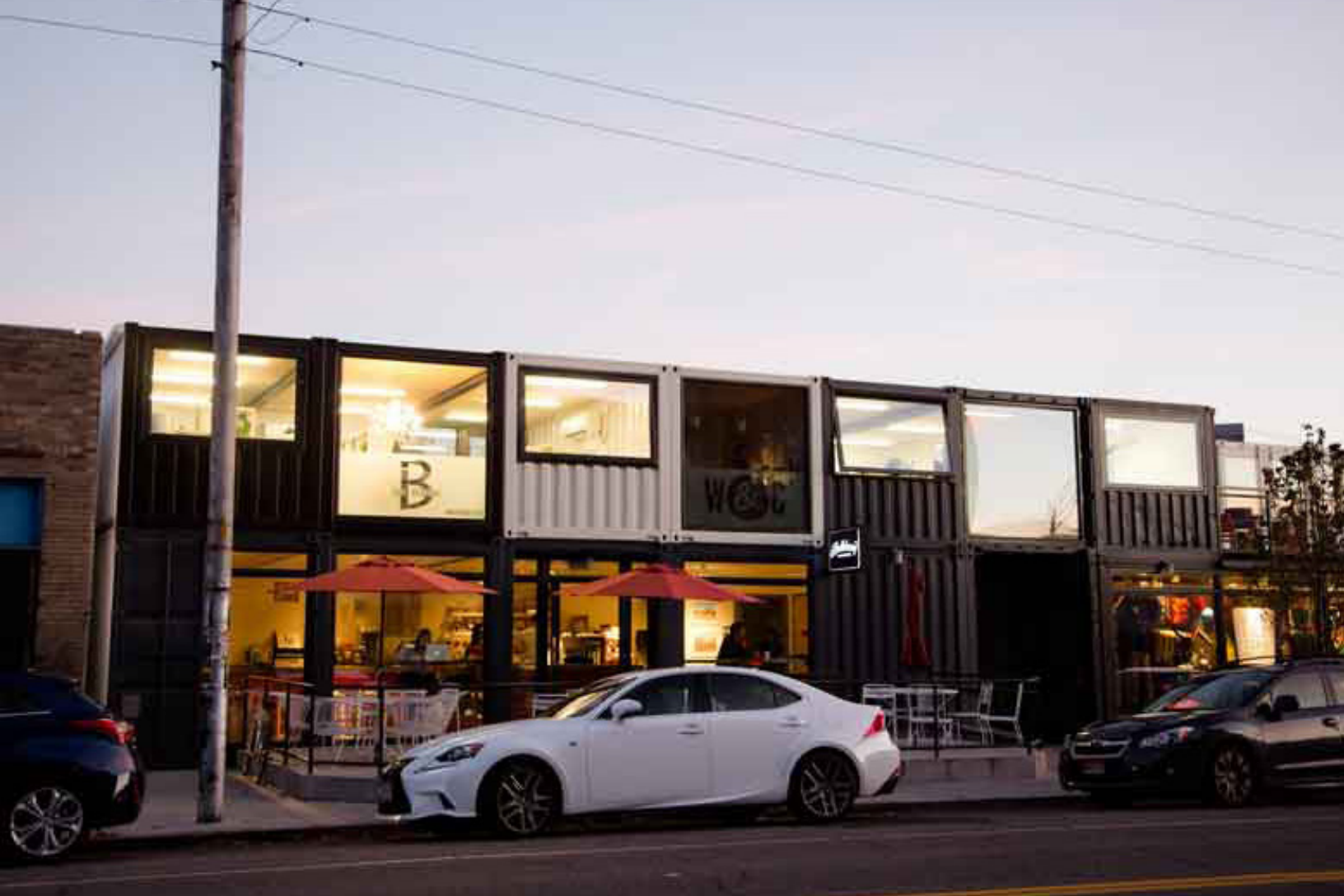
Figure 14 : Photo of 25th & Larimer Building.
