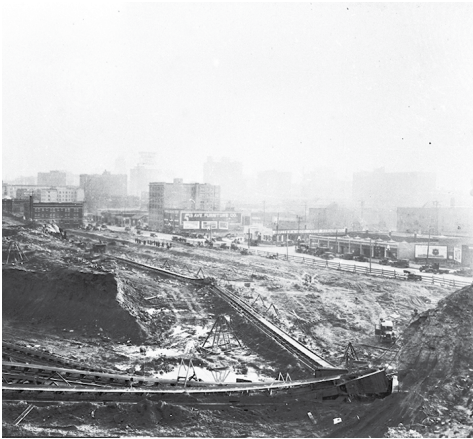
Figure 3.2 (above) Denny Regrade project as seen from 6th and Battery Street in 1929. Courtesy of Seattle Municipal Archives.
