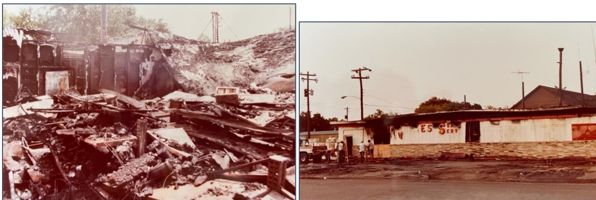
Zackie's after the fire.
