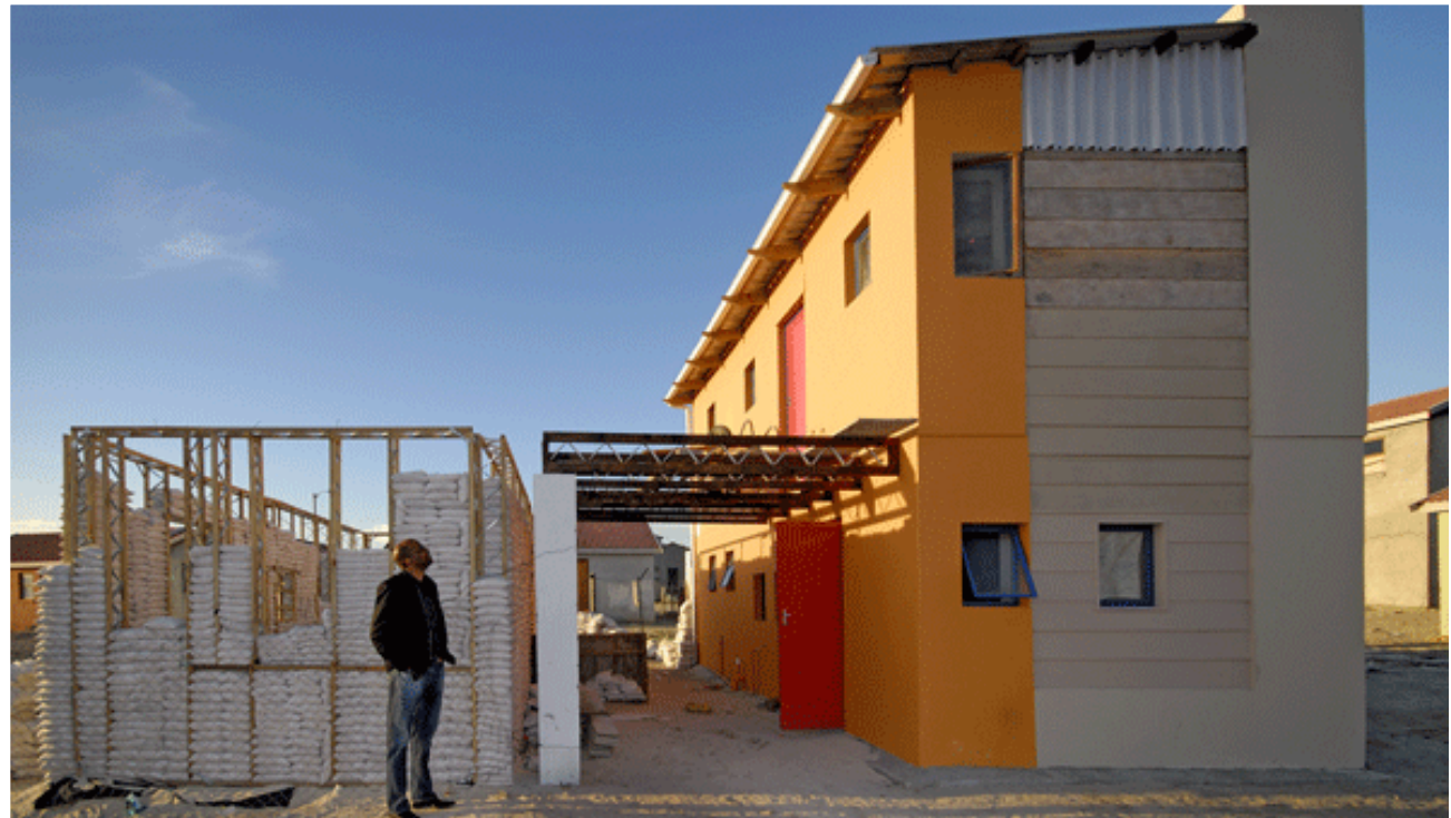
FIGURE 11: SANDBAG HOUSE UNDER CONSTRUCTION 46
