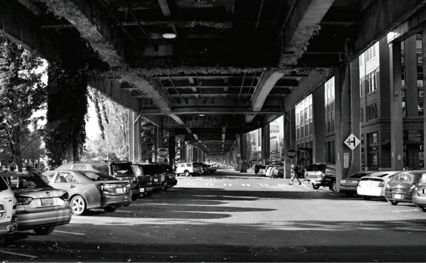
Figure 1.10 Parking Lot under Freeway
