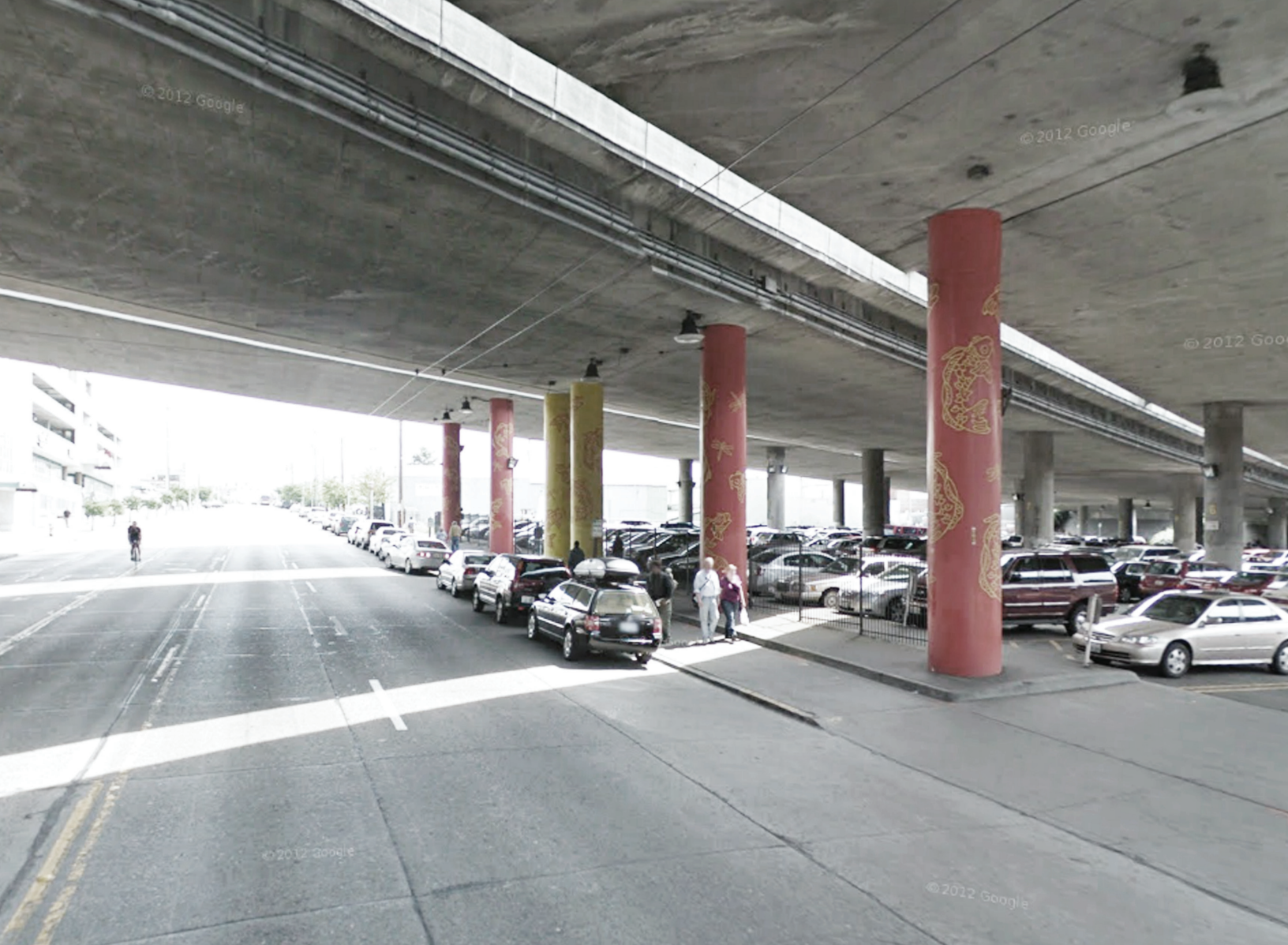
Figure 4.5 The Parking Lot under the Elevated Freeway
