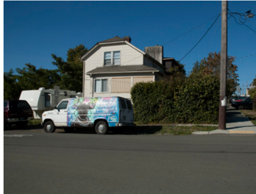
b. Neighbor across Hill Street
