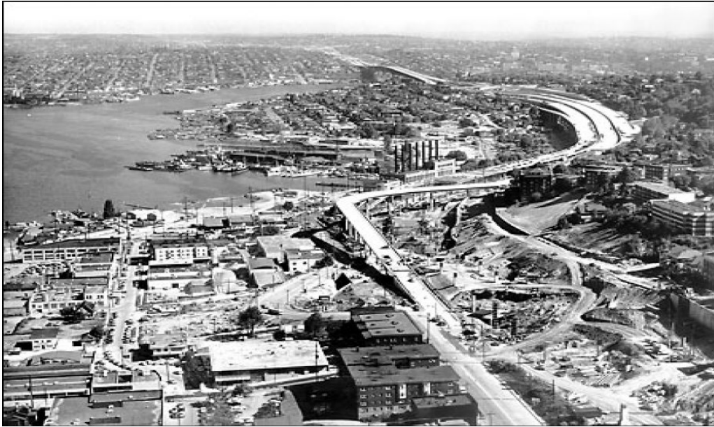
Figure 19: Construction of I-5 spanning the I-5 Colonnade site
