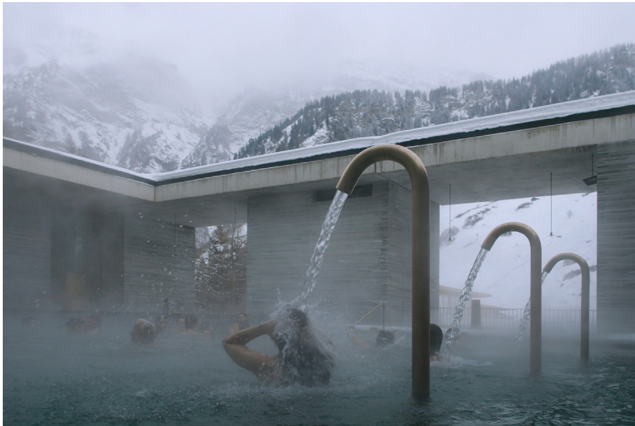
Fig. 4-1: Thermen at Vals, a wellness center in the southern Swiss Alps, reconnects the user to the surrounding mountainside. (Source: Fernando Guerra)
