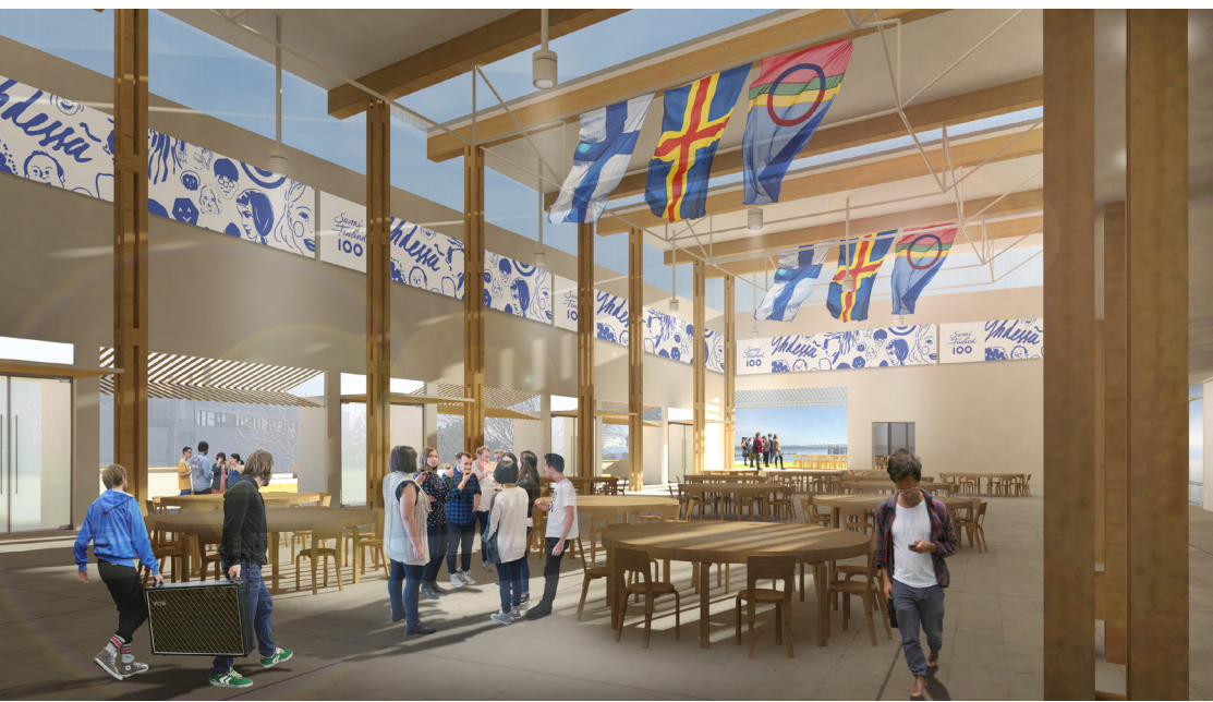
Fig. 7-12: The large flex hall inside boasts skylights that span between heavy timber framing with a king truss underneath, clad in white, giving emphasis to the warmth of the wood.
