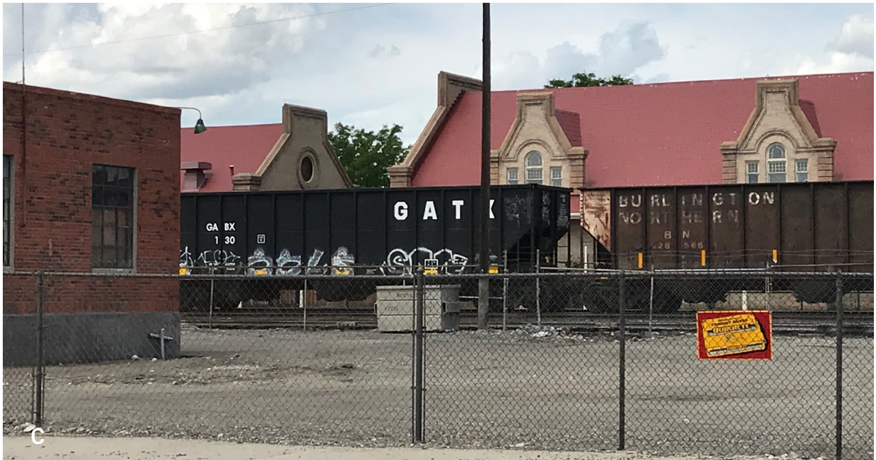
Figure 43 - Back of Billings Depot Figure 44 - Billings Depot from Minnesota Avenue
