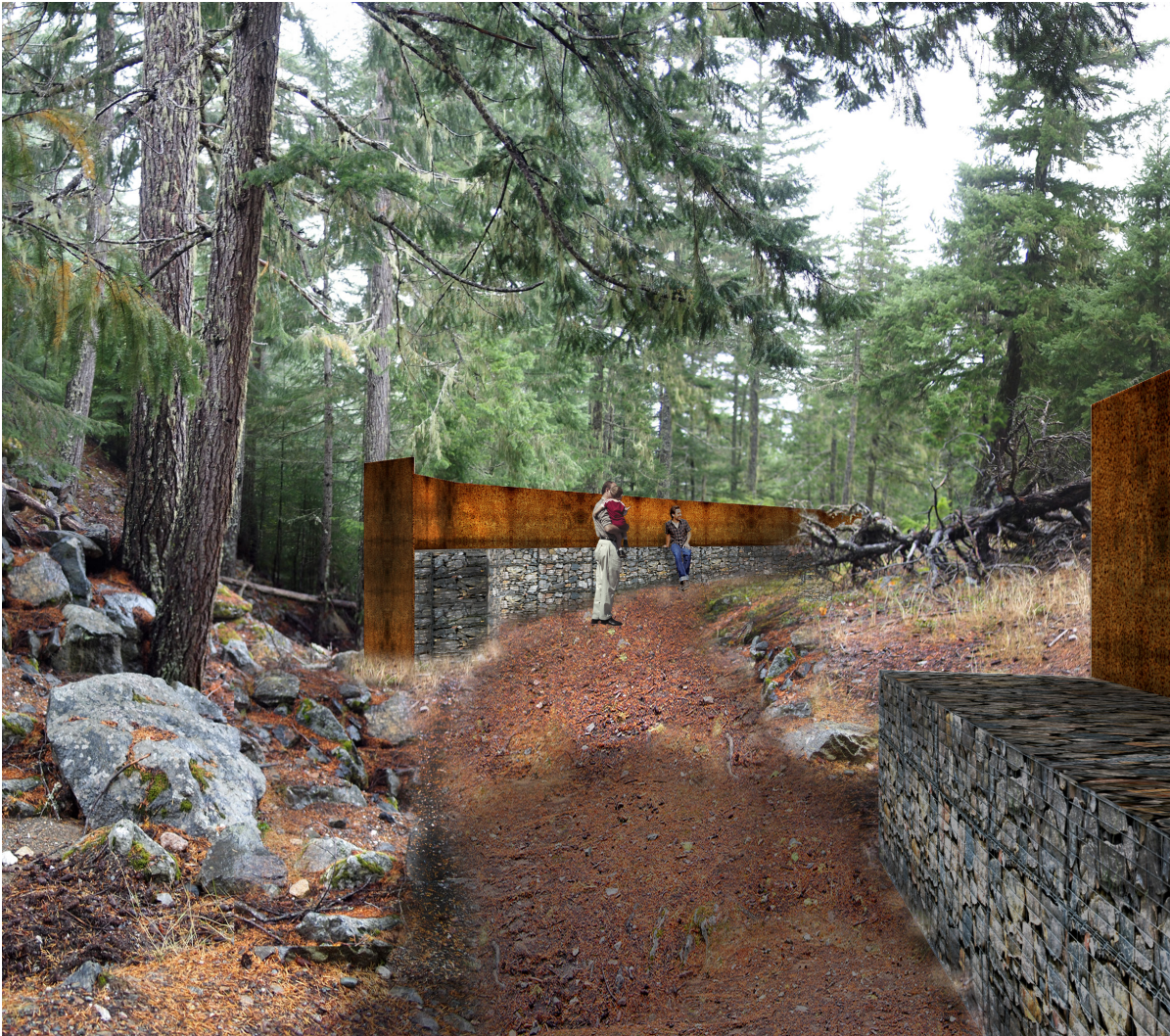
FIGURE 43 Gabion and metal wall
