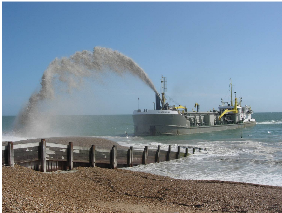
Figure 12. Beach nourishment in progress.
