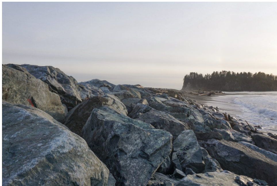
Figure 17. Photo of Rialto Spit Revetment Repair project in La Push, WA.
