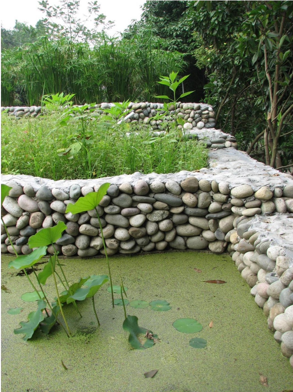
Figure 20. The water treatment system outside Chen's yard. (Photo by Angie McCarrel.)
