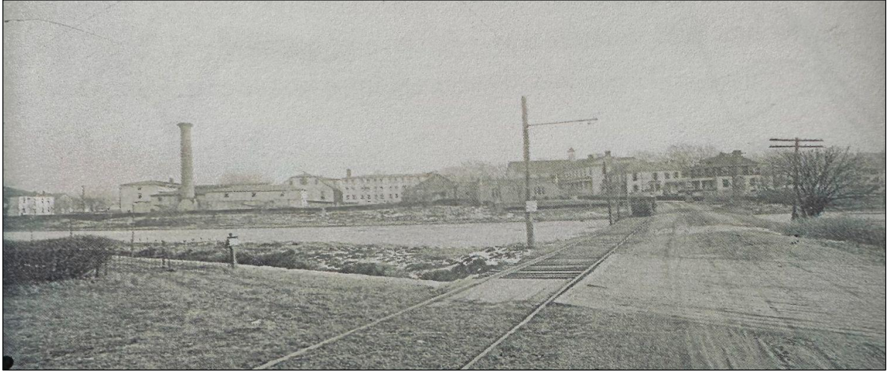
Figure 65: Pratt Avenue Entrance over LeTort Creek, ca. 1910 (Theimer, 2024)
