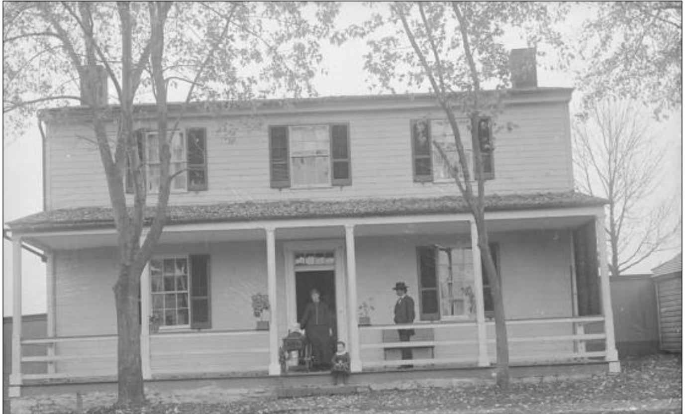
Figure 45: Assistant Superintendent's Quarters, ca. 1880 (Carlisle Indian School Digital Archives, Dickinson College)
