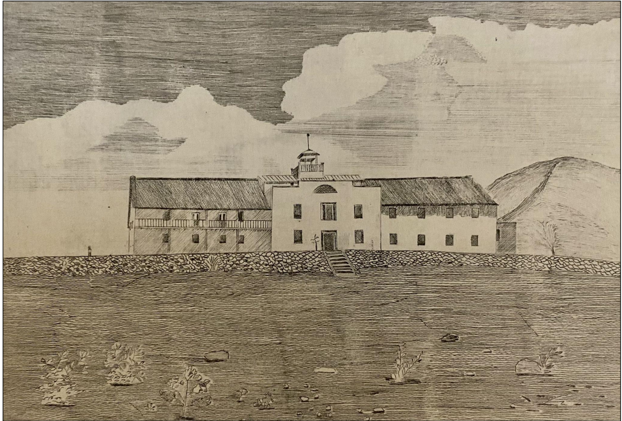
Figure 21: Lahainaluna Seminary Administration Building, 1834 (Hawai‘i State Archives)
