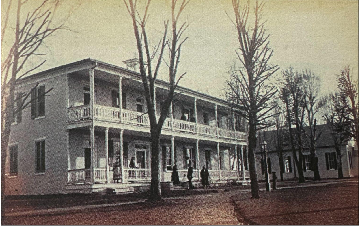
Figure 43: Original Superintendent's Quarters, ca. 1881 (Theimer, 2024)
