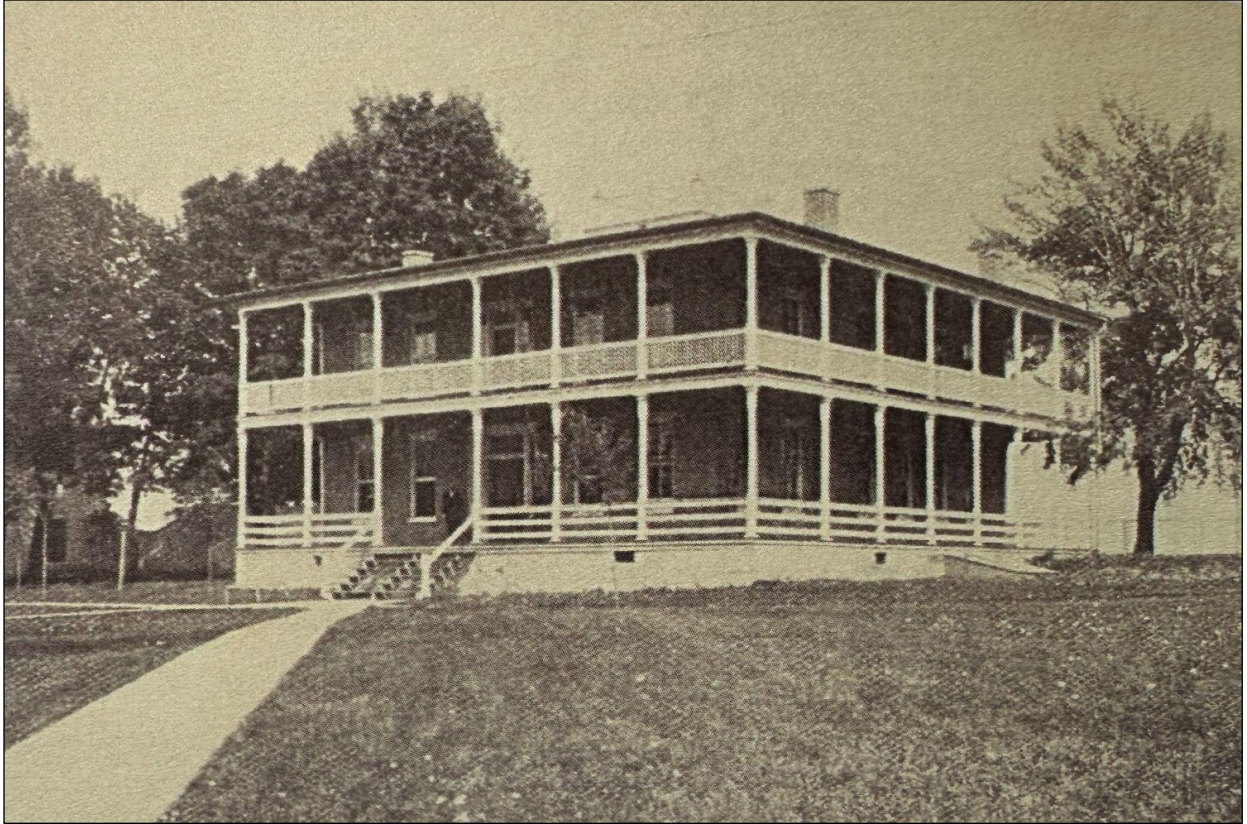
Figure 42: Administration Building, ca. 1895 (Theimer, 2024)
