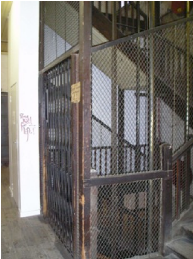
Figure 5-5: Elevator to the top floor...
