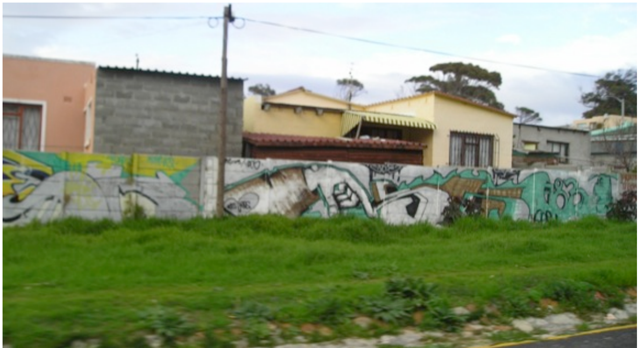
Figure 5-9: Lwandle Township cinderblock houses (2007 photo by author).
