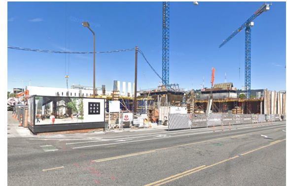
Fig10. Construction site in SLU Image source: Google Street View
