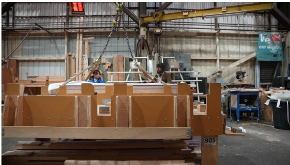
Figure 3-20: Using Crane to Transport the Standard Wall Facing Homelessness
