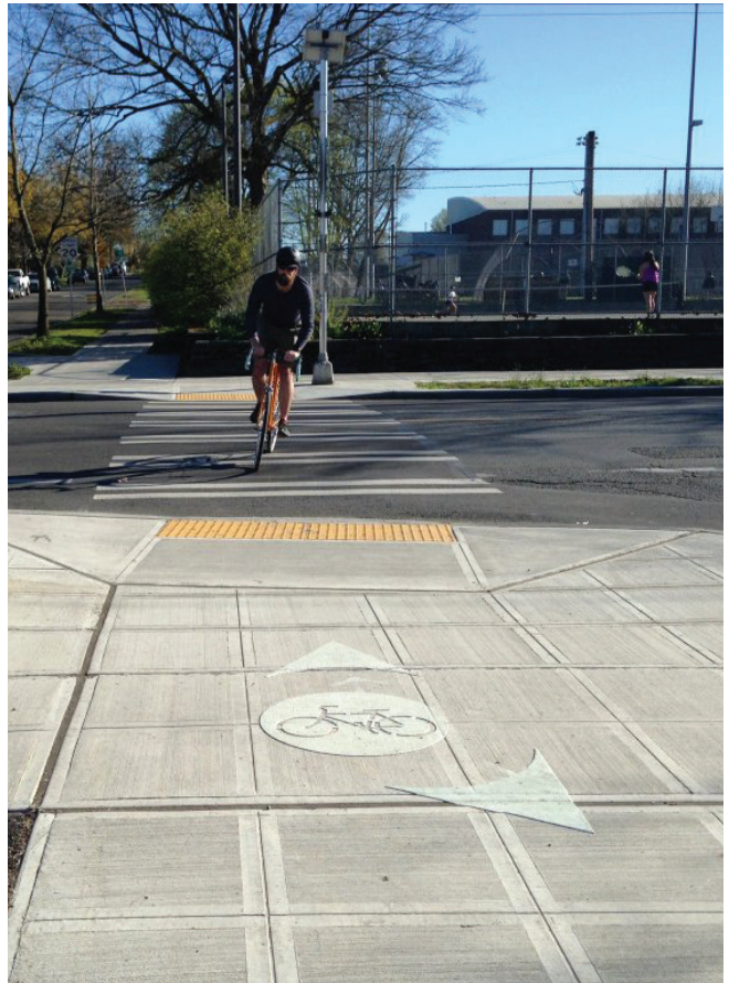
Bike dots help direct bikes as the Central Area Neighborhood Greenway crosses E Cherry St. (image courtesy of SDOT)
