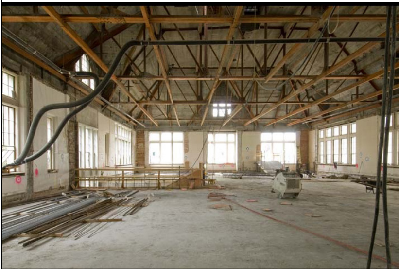
Figure 25: The 2009 renovation retained the structure and historic shell of Savery Hall. Credit: John Stamets, 2008, courtesy UW CPD.
