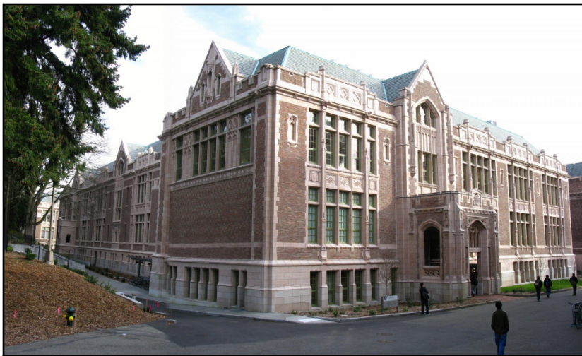
Figure 28: The renovation preserved the exterior shell of Savery Hall. Credit: Mason Contractors Association of America, 2009.
