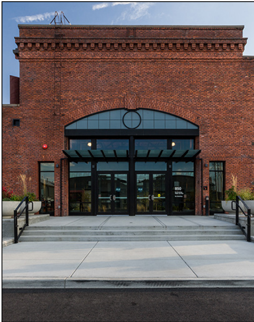
Figure 37: The main entrance of the SIERR Building after it's 2011 rehabilitation is an example of the sensitive interventions completed in the rehabilitation where new construction is inserted into the historic building. Credit: Dean Davis, 2011. Photo courtesy of McKinstry.
