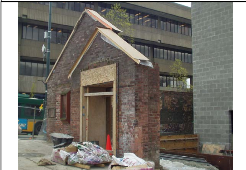
Figure 20: The exterior wall of the historic main entry was retained. Credit: Staff photo, UW CPD, 2008.
