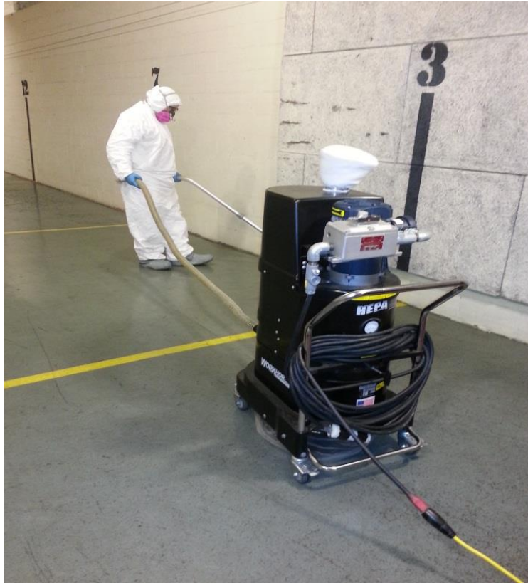
Figure 5 Cleaning personnel using HEPA vacuum cleaner inside the range (Photo by MA Torres).
