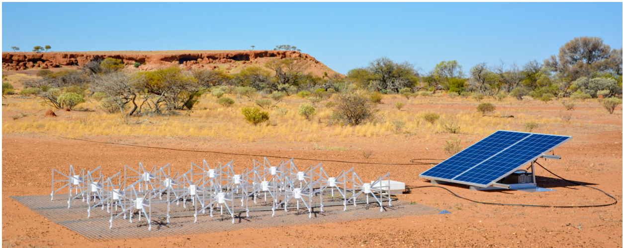
Figure 3.2: An MWA antenna tile, beamformer, and solar panel. The antenna comprises 16 dipoles attached to a mesh screen. They are connected to a beamformer, the small white box to the right of the tile. The beamformer applies delays to each dipole's measurement which effectively 'points' the antenna at some location on the sky. The beamformer then collects the dipole electric field measurements into a single antenna measurement for each polarization. This particular tile is located far from the center of the array, so its beamformer is powered by a solar panel. Image credit: ICRAR/Curtin (accessed from the MWA multimedia archive).
