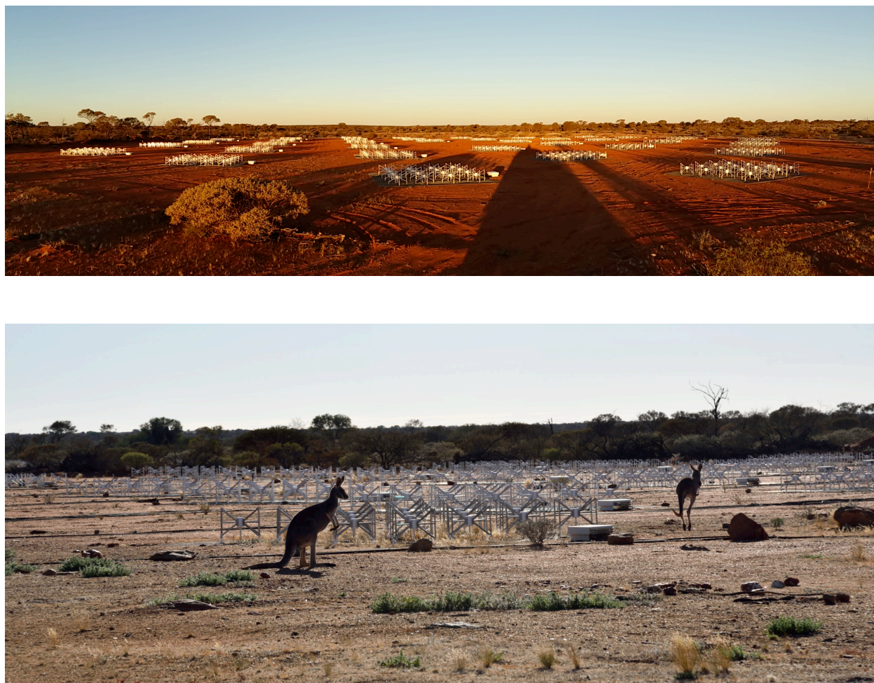
Figure 1.3: Several antenna tiles of the Murchison Widefield Array (MWA), installed at Inyarrimanha Ilgari Bundara , the Murchison Radio-astronomy Observatory. The MWA is located on Wajarri Yamaji Country in Western Australia. The upper image shows a group of antenna tiles arranged in a regular hexagonal pattern. The lower image shows kangaroos visiting the telescope. Image credit: ICRAR/Curtin (accessed from the MWA multimedia archive).
