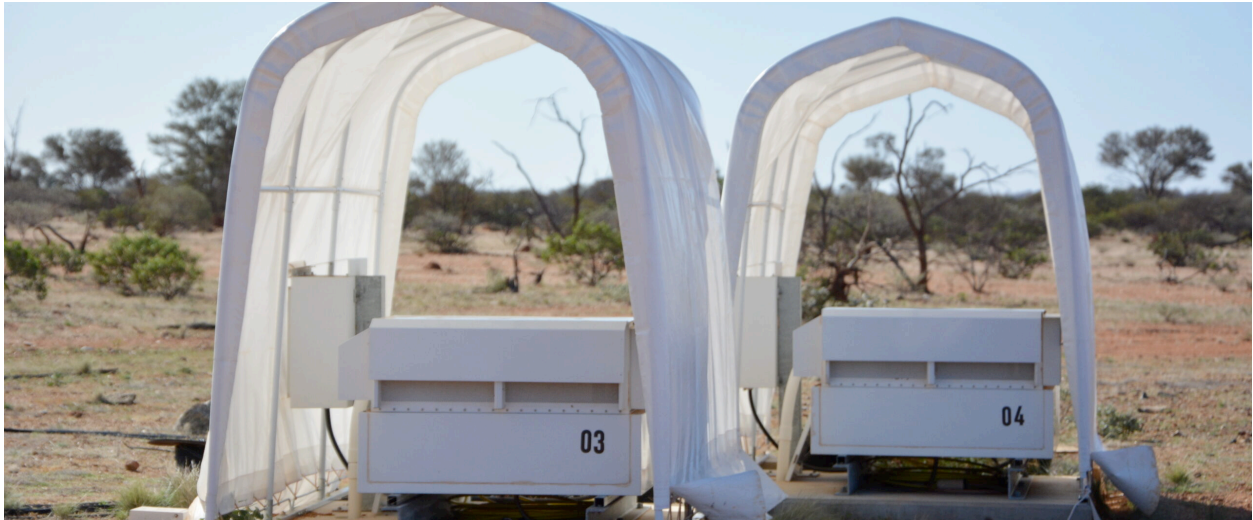
Figure 3.3: Two MWA receivers in sun shelters. Each receiver processes signals from 8 antenna tiles and houses analog and digital signal processing modules. Image credit: ICRAR/Curtin (accessed from the MWA multimedia archive).
