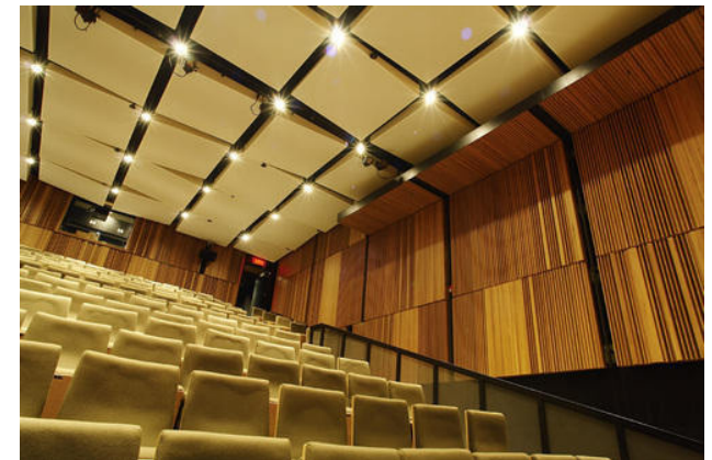
Figure 16 | Specially fabricated sound-absorbing panels, often used in acoustically-controlled environments such as auditoria [Source: WSC Building Materials]
