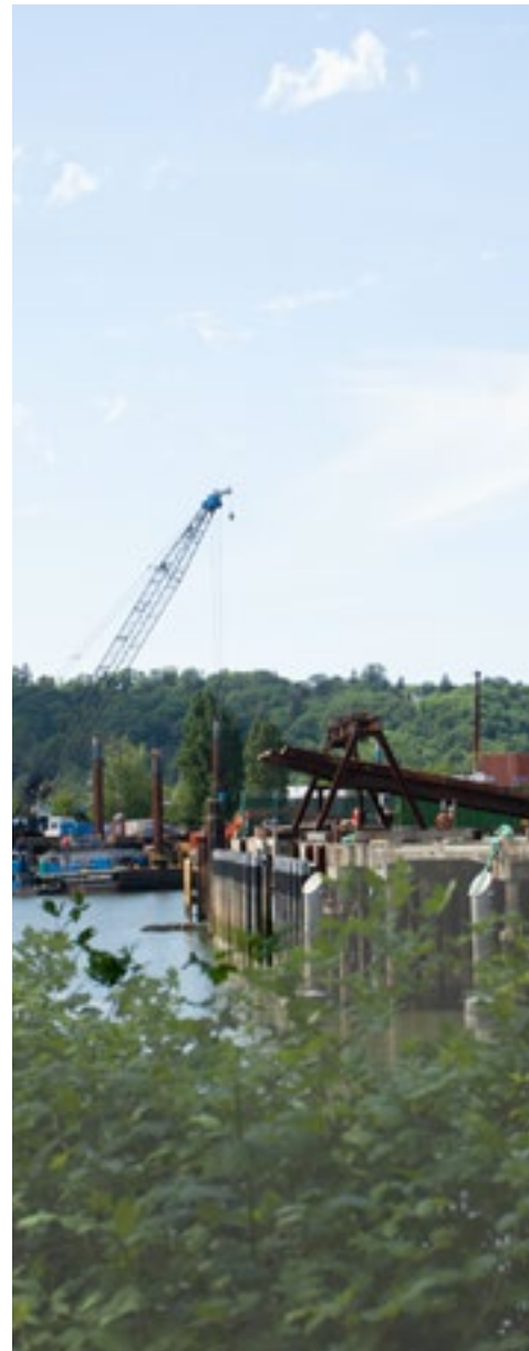
FIG. 8: CONSTRUCTION ON THE RIVER
